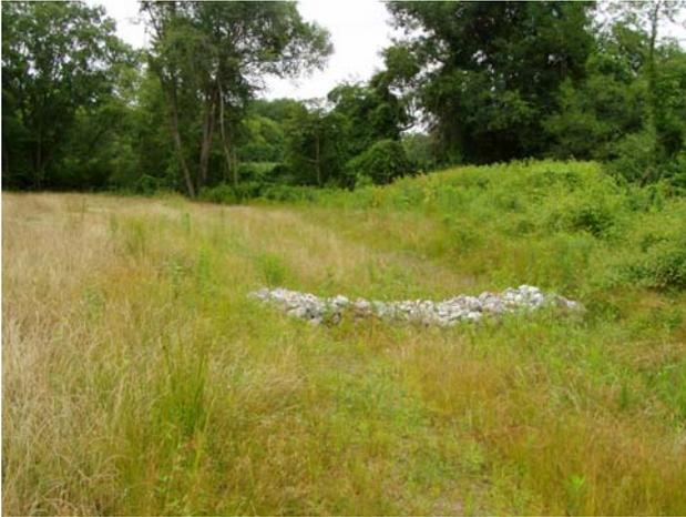
Biofiltration swales convey runoff at shallow flow depths through wide, flat-bottomed swales. They can be very effective in removing Total Suspended Solids (TSS) and adsorbed metals, although less effective in terms of decreasing the amount of nutrients contained in water.
