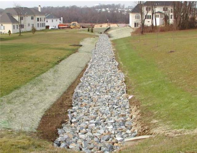
Most Green Technology BMPs incorporate infiltration as part of the treatment process. Specific infiltration facilities include infiltration trenches. Infiltration trenches located in swales provide additional wetted surface area and storage volume, and often they can be designed to penetrate shallow impermeable soil profiles to recharge deeper soil horizons.
