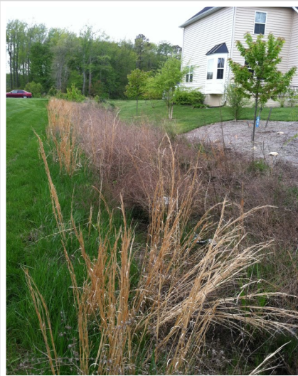
Bioswale with Native Grass
